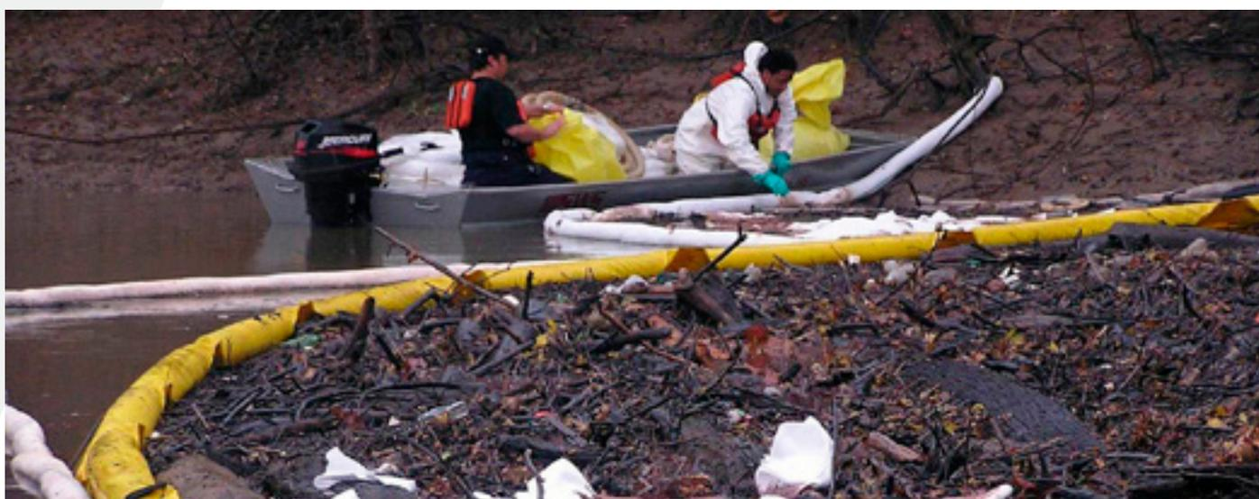
Solid Flotation Boom, height: 254-1067 mm (10-42 in)
