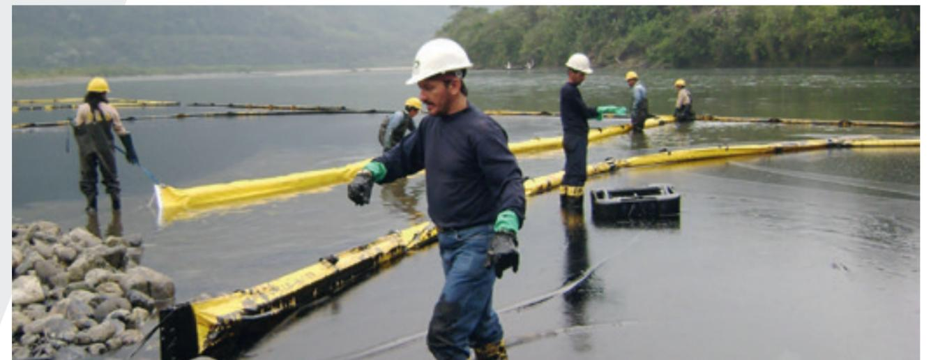
Solid Flotation Boom, height: 360-920 mm (14-36 in)
