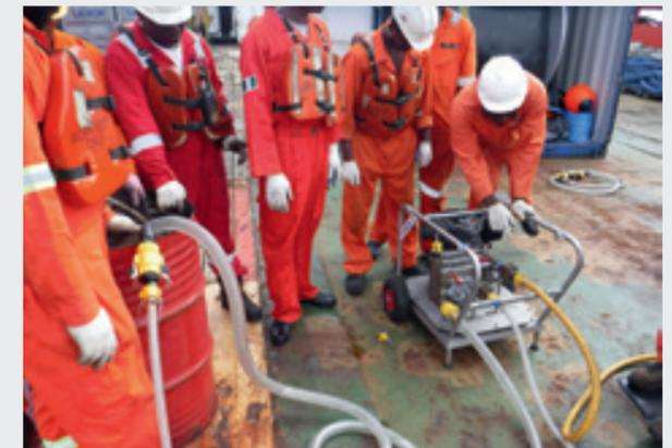
Deployment of dispersant system onboard vessel
