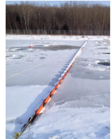
Baffles deployed in ice conditions
